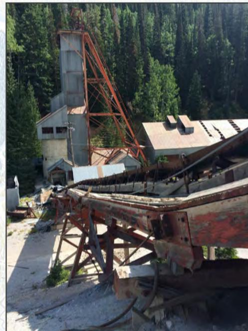
This enormous dump is the result of a futile exploration by the Silver King Coalition into barren ground. The conveyor took the waste rock from the shaft and tunnel system below and deposited it here on the dump.
