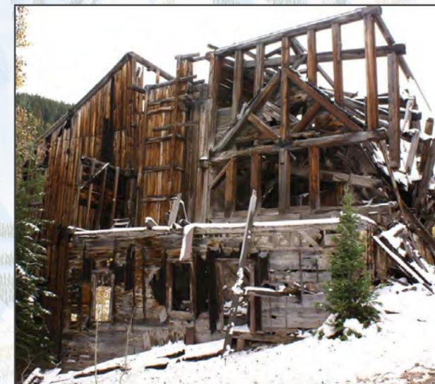
The California-Comstock stamp mill has been deteriorating since 1917 when it was last remodeled. It could process 150 tons of ore per day and was operated by very few men. Solon Spiro's Tunnel lies 1700-feet underneath this. It is connected underground to the Thaynes Shaft via the West End Tunnel where skiers used to ride the Skier Subway to alight at Thaynes Lift in the early days of Treasure Mountain Resort.
