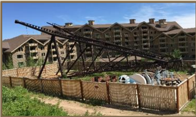
Daly West Headframe - Collapsed in 2015
