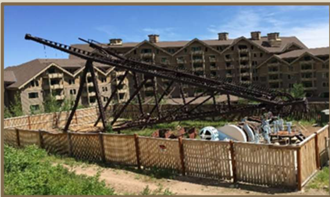
Daly West Headframe - Collapsed in 2015
